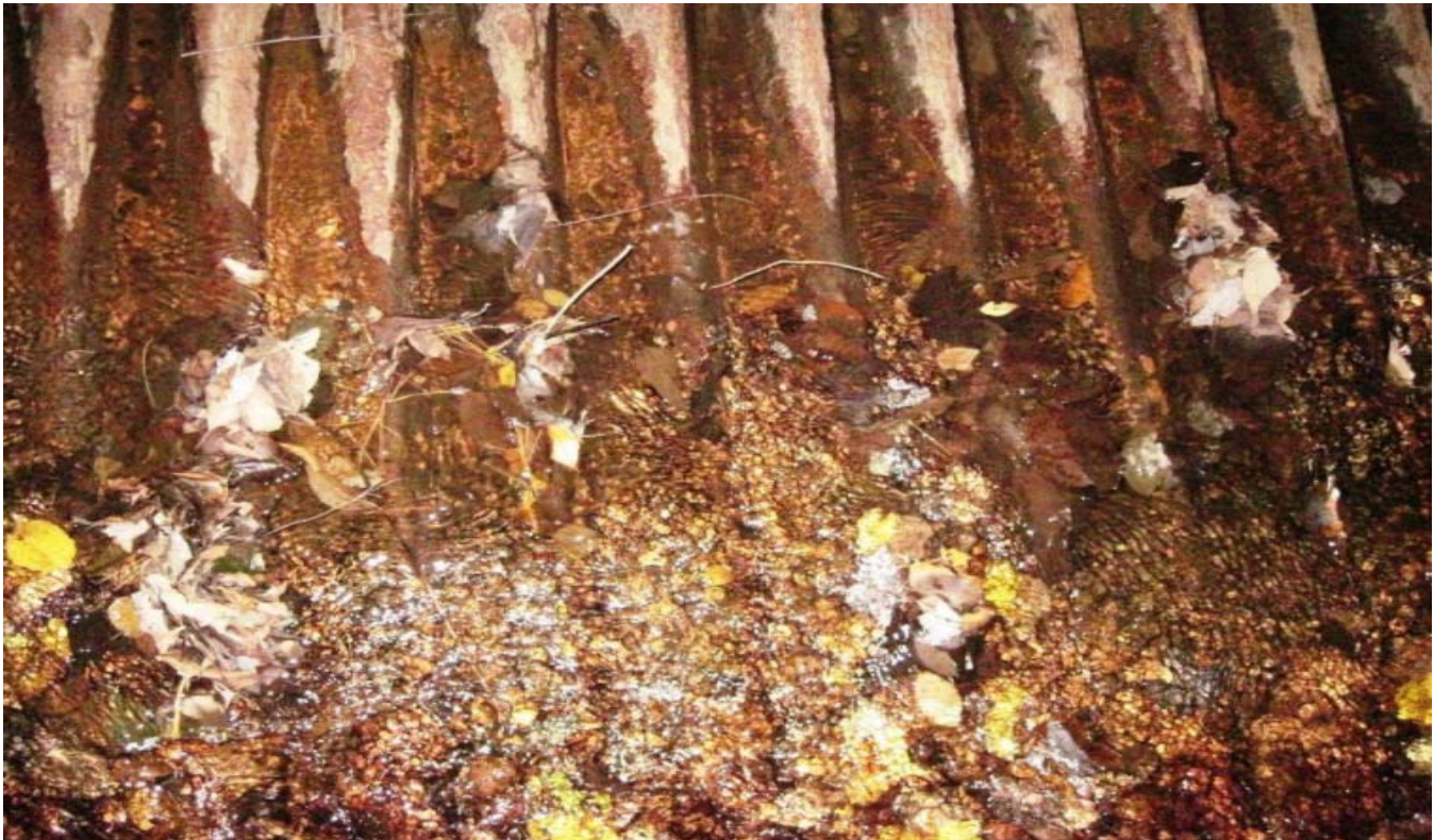
Deteriorated Invert
